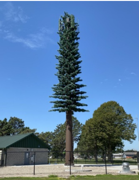
Stealth Cell Tower Source: Marvin Planning Consultants
